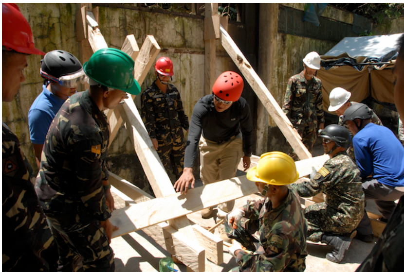
Members of the Philippine Armed Forces put what they learned to use. The construction is called a split sole racker and is meant to stabilize a weak wall. Camp Lapu-Lapu, Cebu, Philippines, Mar. 3, 2014. (U.S. Air Force Photo/SrA Orlando Corpuz)
