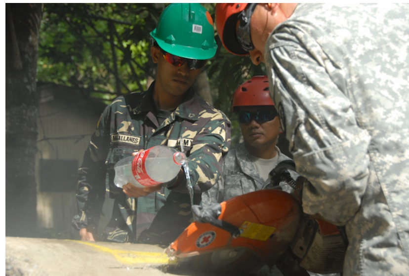
You got to use what you got. Water is poured from a coke bottle onto a saw to keep the blade from overheating and to keep the dust down. Camp Lapu-Lapu, Cebu, Philippines, Mar. 10, 2014. (U.S. Air Force Photo/SrA Orlando Corpuz)
