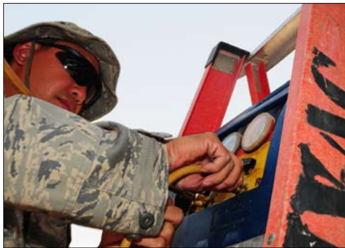
Airman Christopher Aurio, 386th Expeditionary Civil Engineer Squadron Heating, Ventilating, and Air Conditioning apprentice, prepares to recover refrigerant from a packaged air conditioning unit at an undisclosed location in Southwest Asia Aug. 5. Airman Aurio is deployed from the 154th Wing, Hickam Air Force Base, Hawaii. (U.S. Air Force photo/Tech Sgt. Tony Tolley)
