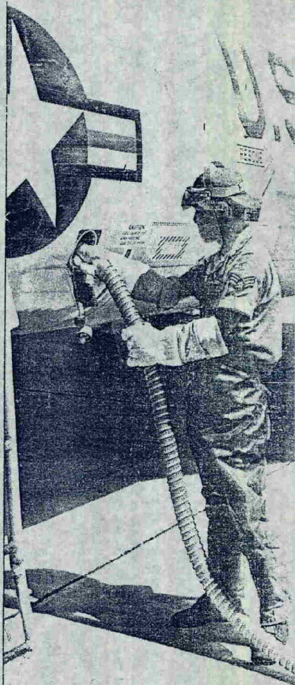
SGT. SAITO, ONE OF THOSE HARD WORKING UNSUNG HEROES OF THE FLIGHTLINE FILLS THE LIQUID OXYGEN TANK OF A DEUCE. THE OXYGEN WILL BE CONVERTED TO A GASEOUS STATE IN THE AIRCRAFT AND USED FOR PILOT BREATHING.
