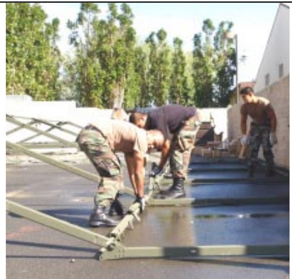
154 SVF members assembling a temper tent prior to moving to their deployed site at zone F.
